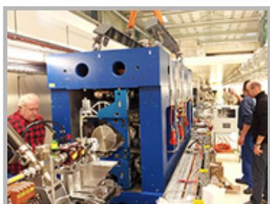
**Installation of SwissFEL Undulator Prototype in the Injector Test facility.**
